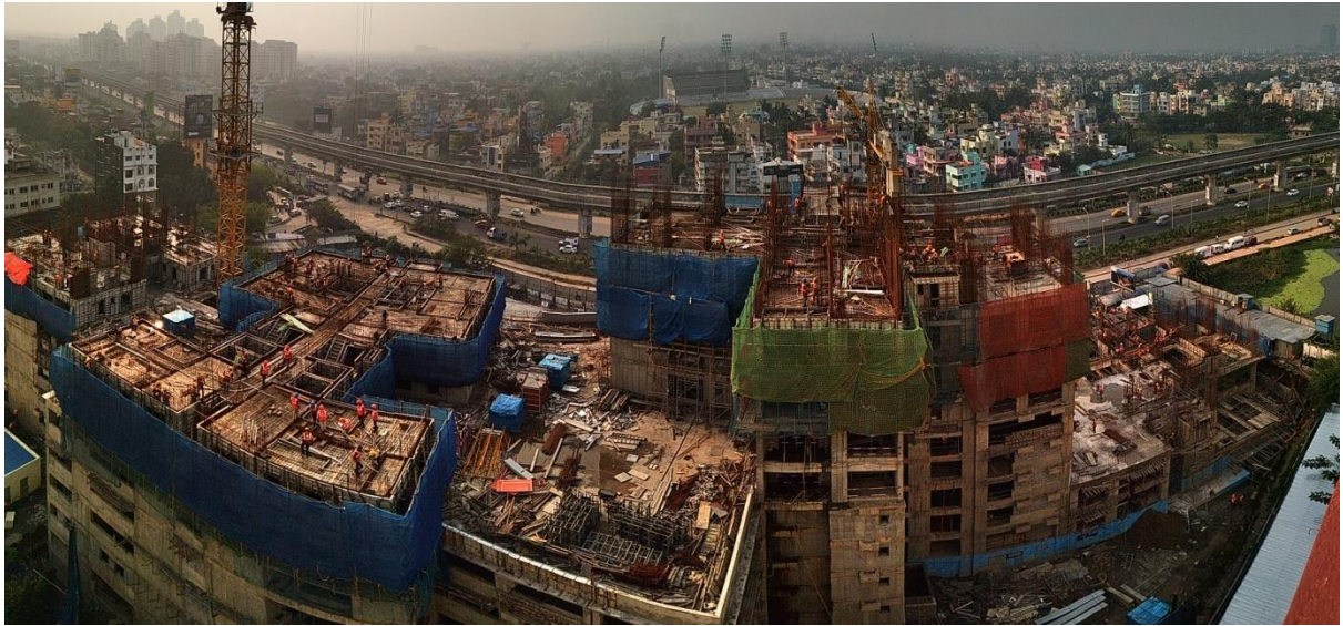
AVIDIPTA PH – II Construction going on
